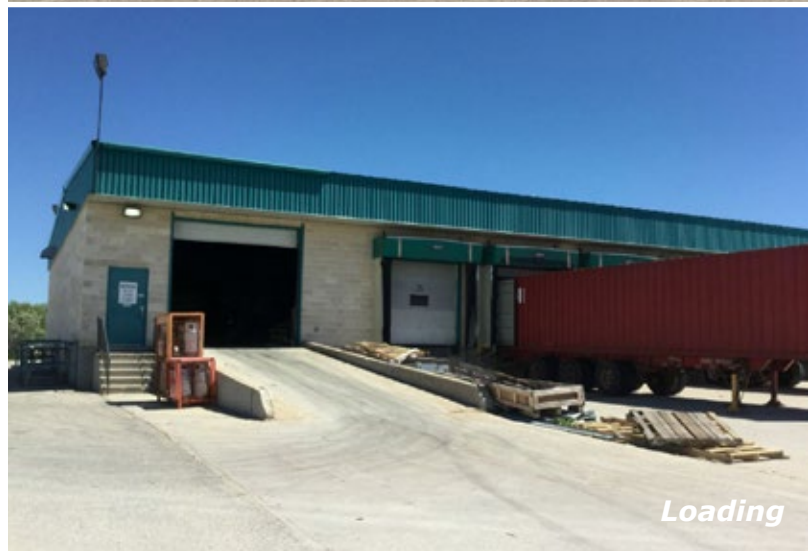
Truck & Trailer Parking
